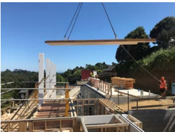
Figure 2 Tag lines attached to panel.
