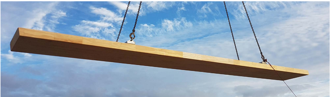
Figure 1 Tag lines attached to panel.
