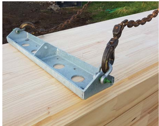
Figure 3 Bolt on lifting brackets.
