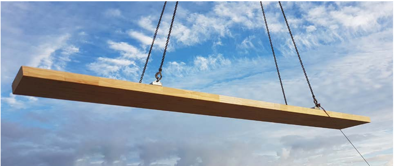
Figure 3 Bolt on lifting brackets.
